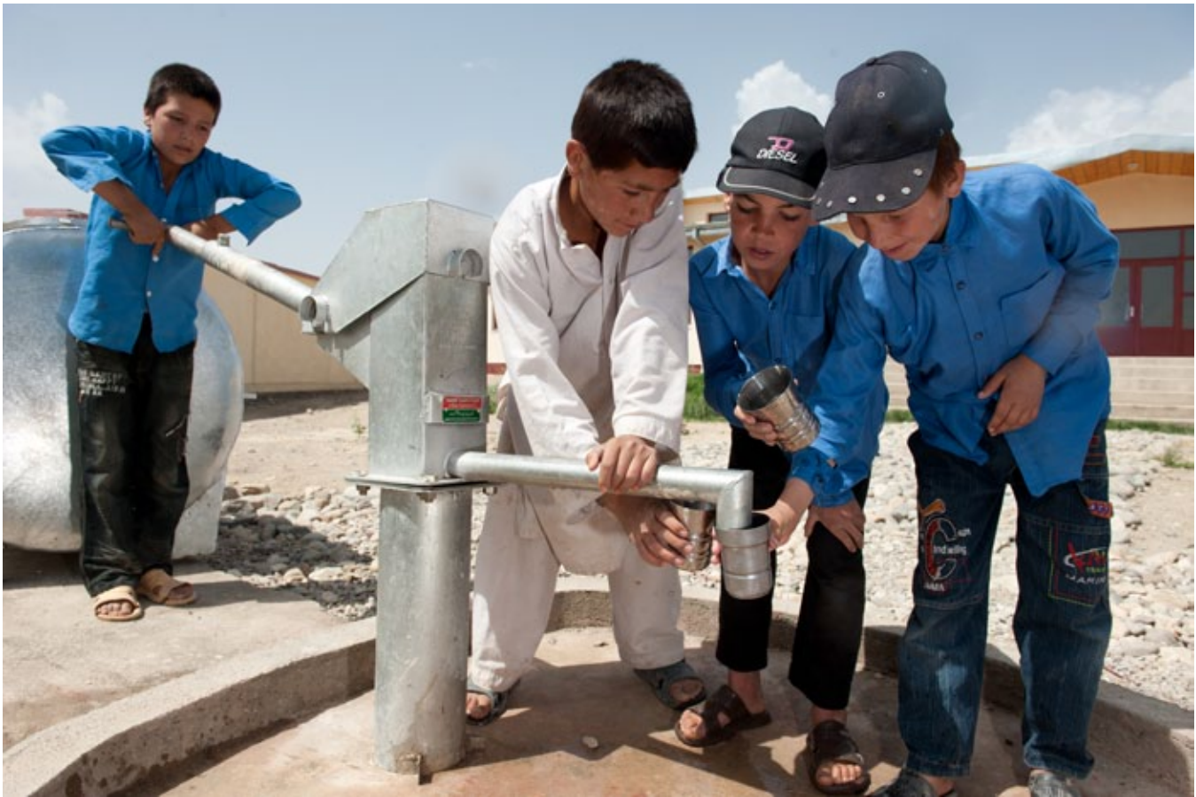
Boys taking water from the school's new well in Guldara District just outside Kabul. The well was completed three weeks earlier with the support of Save the Children — funded by the Khalifa Bin Zayed Al Nahyan Foundation. Photo Credit: Mats Lignell
